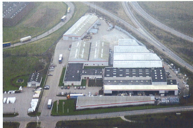
JUMBO Stillads is Denmark's leading supplier of scaffolds, ladders, and working platform lifts
