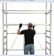
Mount 4 horizontal braces between the railway frames. Now move your platform to the desired height
